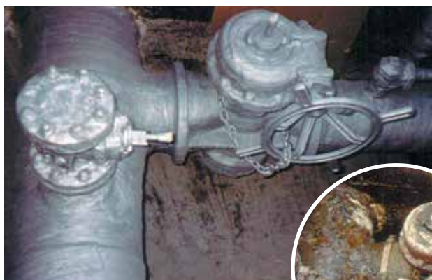
Trenton Wax-Tape® brand anticorrosion wraps, such as Wax-Tape #2A self-firming anticorrosion wrap, excel in limited-access situations, such as vaults, where surface preparation is difficult.
